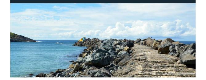
Across the eastern seaboard of Australia, breakwaters and training walls have instigated fundamental perturbations to coastal and estuary processes. This has induced long-term changes to foreshore alignments, tidal currents, tidal planes and marine ecologies, with significant consequences. These effects can be seen right along the NSW coast of Australia, where breakwaters and training walls have been implemented.
